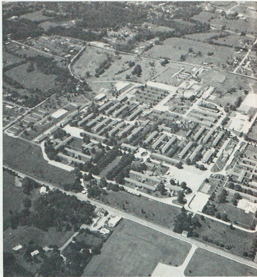
Valley Forge Christian College of the Assemblies of God campus in Phoenixville, Pa., a 77-acre tract with 70 buildings. It formerly was the Valley Forge Army Hospital.
