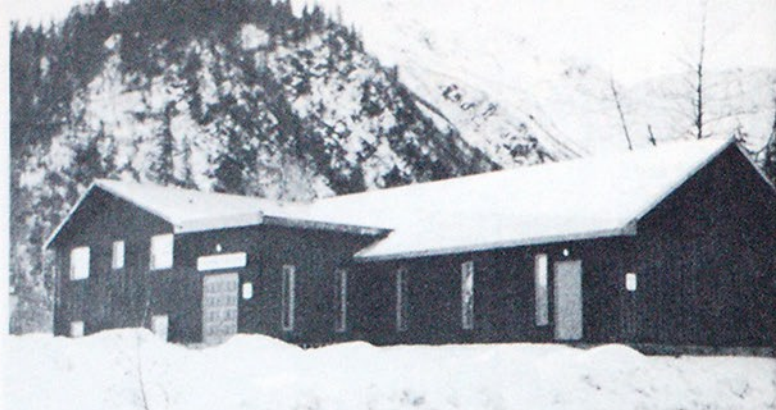
This new building was dedicated by the congregation of the Assembly of God, Seward, Alaska, in January.
