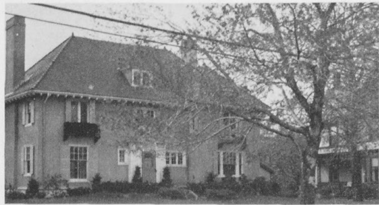
This house serves as headquarters for the Boston Teen Challenge.
