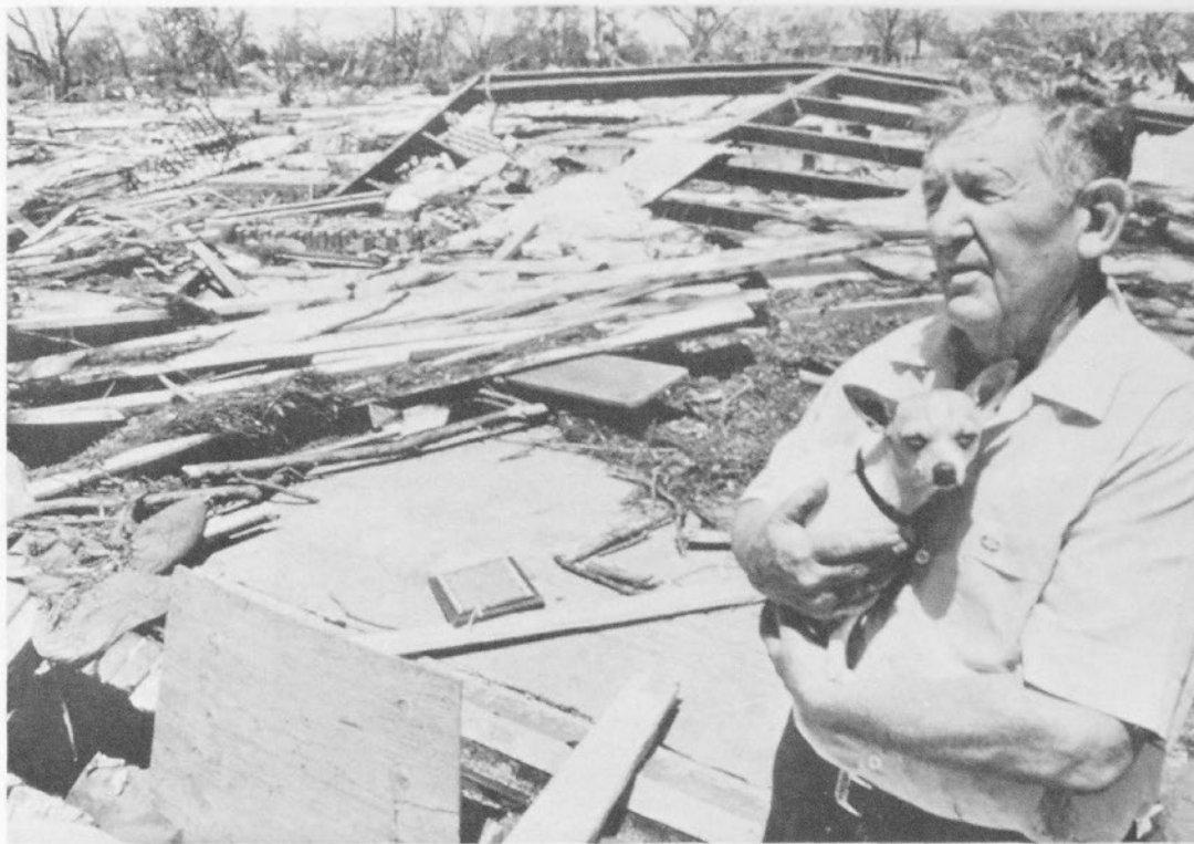
He left and lived. Earl B. Matthews stands amid the rubble that is all that remains of the apartment building at Pass Christian, Miss., where 23 died during hurricane Camille. (AP wirephoto)
