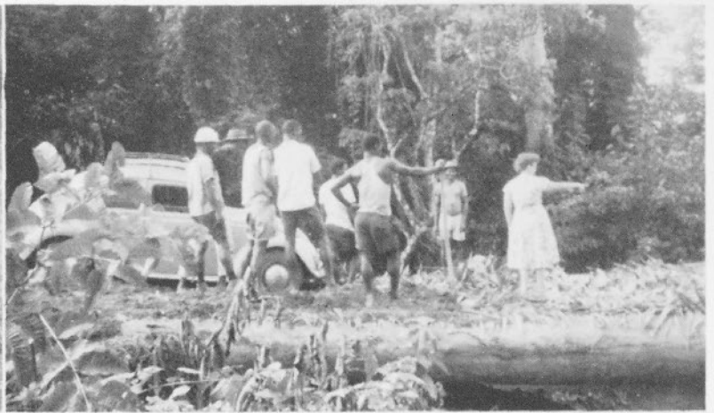
A side trip reaches a nearby village during delay while workers fill up gaps between logs so the car can cross the bridge.
