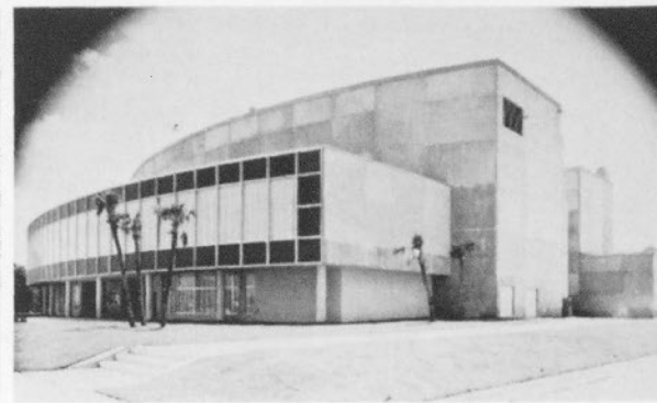
Municipal Auditorium, Panama City, Florida
