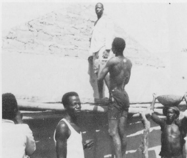
Mud brick walls were plastered to make them rainproof.
