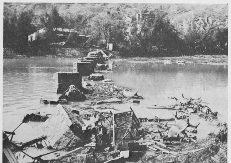
The concrete foot-bridge connecting the school with the road was demolished. Bodies of pigs litter the banks as the river recedes.
