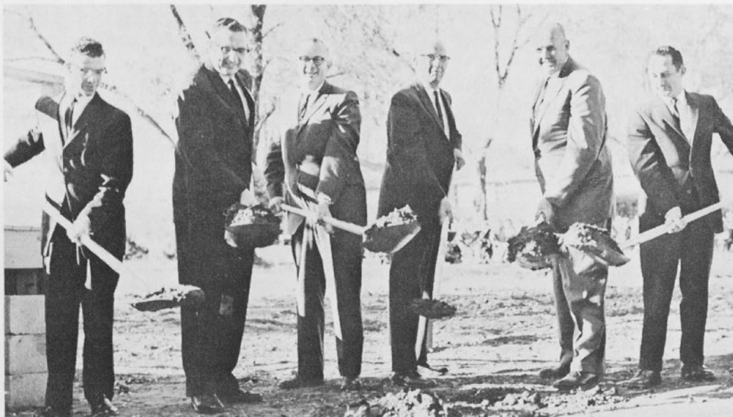
Participating in the groundbreaking ceremony were (left to right): Glenroy Shedd, president of Evangel College student body; J. Robert Ashcroft, president of Evangel College; Thomas F. Zimmerman, general superintendent of the Assemblies of God; Guy Basye, member of Evangel College board of directors; Al Rediger, president of the Council of Evangel College; and Jim Teuber, vice-president of Evangel College Alumni Association.
