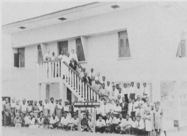
Assemblies of God headquarters building in Enugu, Nigeria
