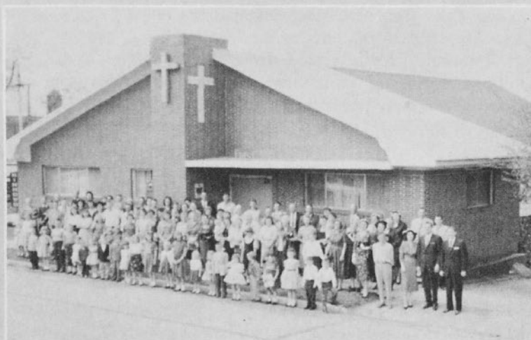
MINDEN, LOUISIANA—Since Leslie E. Hunter Jr. became pastor, First Assembly has added this beautiful and commodious new front to their building. This photo was taken during a recent revival with Evangelist Jack Pruitt of Fort Worth, Texas.
