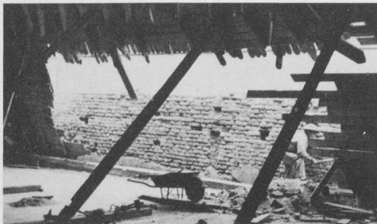
Concepcion Assembly heavily damaged by earthquake
