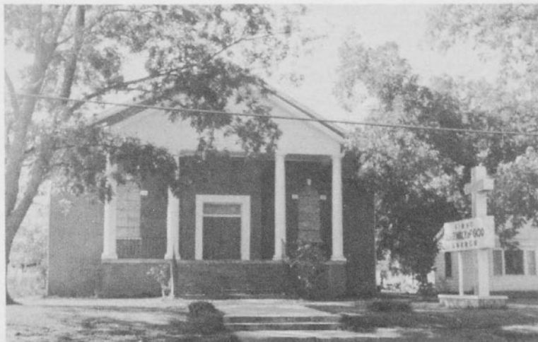
ENTERPRISE, ALA.—First Assembly, organized in 1914, now worships in this new 500-seat church which has Sunday school facilities for 400. Howard P. Trawick has been pastor since 1951.
