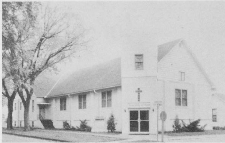
OSKALOOSA, IOWA—The Assembly here has just finished remodeling its church. The auditorium seats 450 and there are 22 Sunday school rooms. Max Johnson is the pastor.
