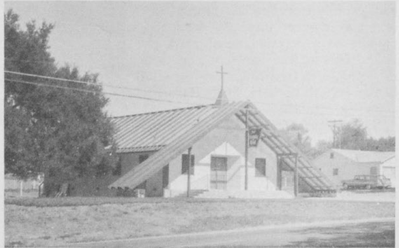
ATASCADERO, CALIF.—The Assembly of God in this little town was remodeled inside and out. Pastor H. P. Wilde, Jr. and his congregation plan to add new classrooms in the near future.
