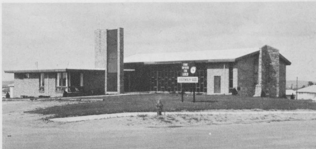
ROCHESTER, MINN.—The Assembly here is thirty years old. The present edifice, however, is new, having been erected since O. E. Carter became pastor. The T-shaped brick veneer and stone structure was designed by A. V. Gustafson, regional architect.
