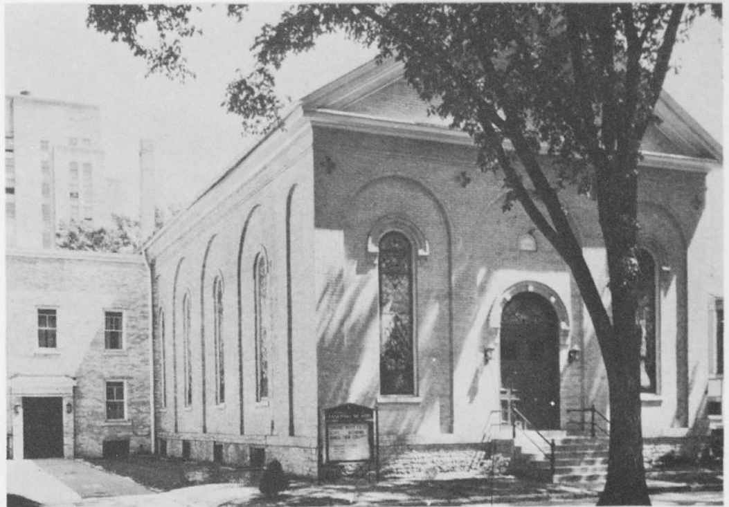
FIRST ASSEMBLY REMODELED AT RACINE, WIS.
