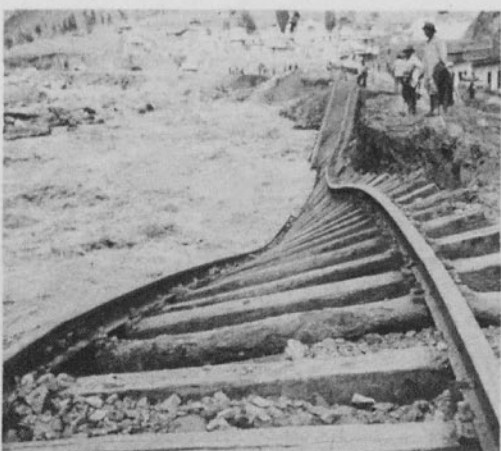
Path of river along the side of sagging railroad track. At this point the angry swelling river went out of bounds and billowed over the mountain town of Matucana.
