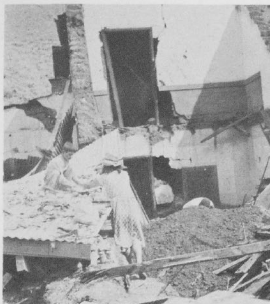
Only a few houses of cement and brick withstood the waters. Others of adobe brick were dissolved and washed away.
