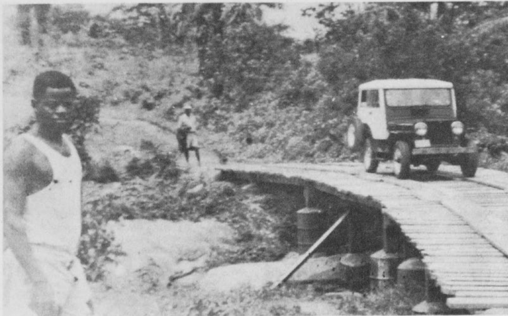
Recently constructed seventy-foot bridge that enables the missionaries to cross to the Firestone plantation.
