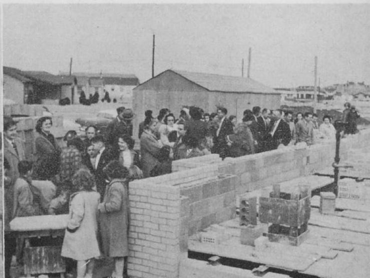
Members inspect construction progress on their new church at 4909 East Monroe, Wichita.
