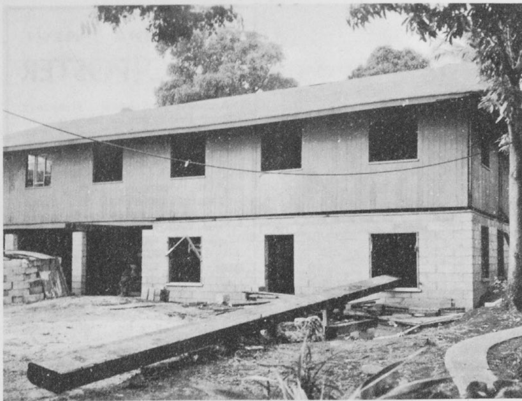
ALOHA BIBLE INSTITUTE DORMITORY IN PROCESS OF CONSTRUCTION
