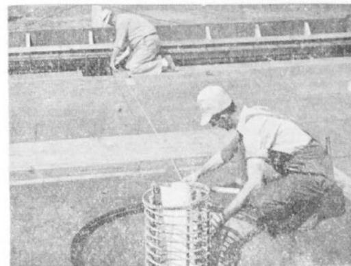
With the figures in mind as the blueprint calls for them, careful measurements must be made. Everything must measure out to the fraction of an inch. The workman in the foreground is in the section over the top of a pillar. Notice the circular reinforcing steel bars protruding from the pillar.
