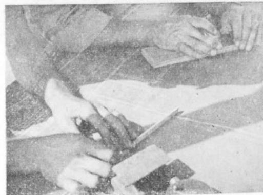
Accuracy is the important thing! One of the foremen and his helper carefully study the blueprints in preparing the layout for a section of the floor before the concrete is poured.
