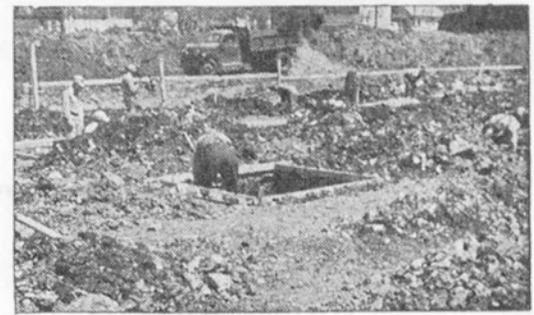
Workmen dug the footings with pick and shovel in preparation for the concrete foundations which will carry the weight of the great presses.
