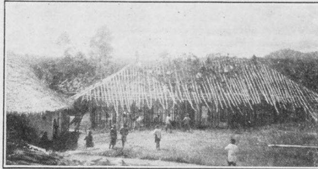
A new dormitory for the Bible school in Feloka, Liberia. All the material is gathered from the forest and used in its crude form. The workmen are tying long bamboo sticks crosswise to the roof sticks. The thatch is then held in place with tie-tie (bush rope).
