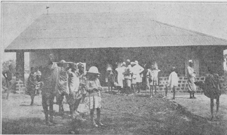
The new chapel and school building in Yendi, Gold Coast. There is a real need at the present time for a competent school teacher to be sent to the Gold Coast in order to assume the supervision of the school work. The government provides equipment and the acquiring of the supervision of the local schools involves concessions in the district for gospel ministry. If we do not take the opportunity others will, whose doctrines we might not approve. Let us take the opportunity and give them the full gospel message. Unlimited freedom is given the teacher in regard to religious instruction in the schools.
