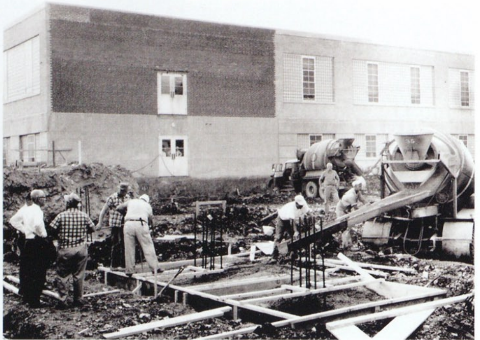
Construction workers pouring the foundation for the new administration building, August 12, 1960. The 2-story printing plant, constructed in 1949, can be seen in the background.
