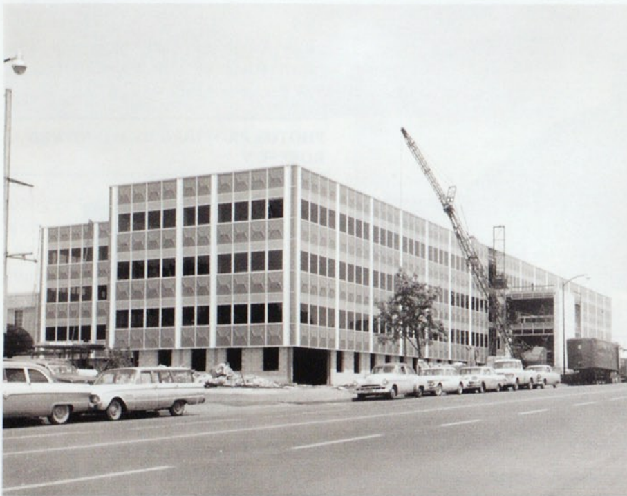
The new administration building nearing completion in 1961.
