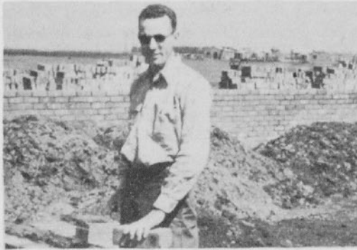
... Vernon Pettenger lays the bricks
