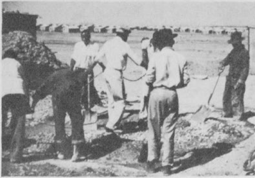
Christian men help mix concrete
