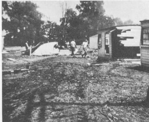
This was the scene along the camp road after the waters had receded four days after the flood. These cabins were part of the 13 destroyed by the flood.
