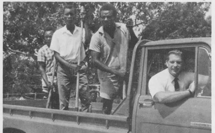
Douglas Blue, MAPS volunteer, works with Congolese Christians on the construction of the new church in Kinshasa, capital of Congo.
