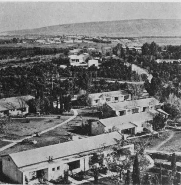
The residents live in modest apartments.
