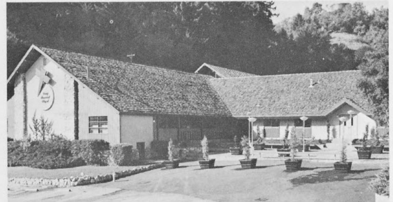
New addition to Craig Memorial Chapel at Bethany Bible College in Santa Cruz, Calif., was dedicated recently.
