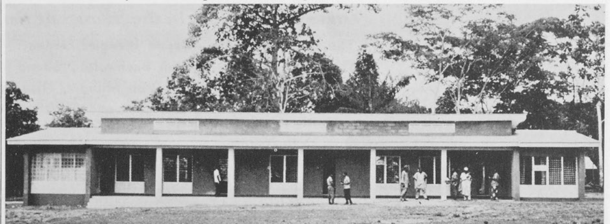
This is the first completed building for Western Nigeria Bible Institute.
