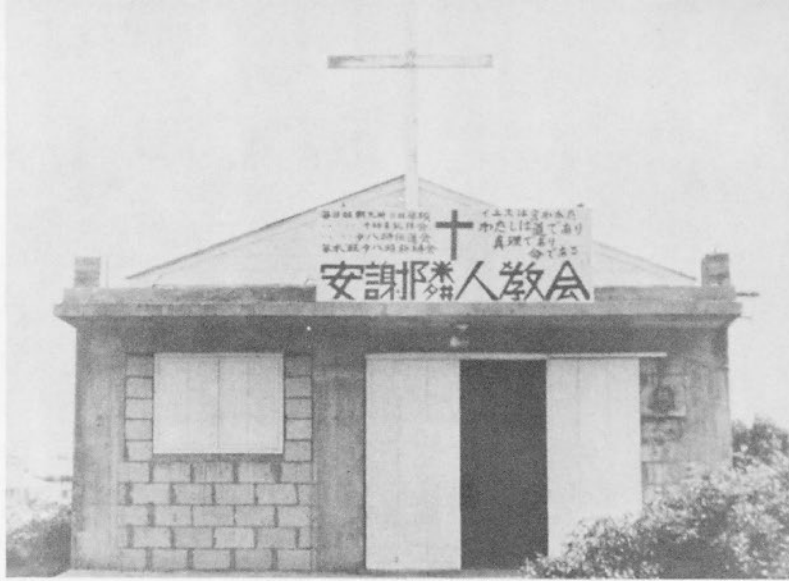
The church at Aja, Okinawa, is made of concrete blocks to withstand the many typhoons which lash the island.
