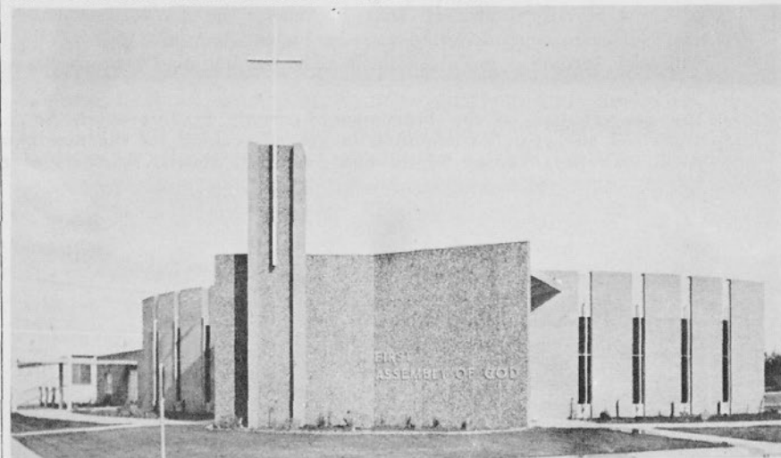
The First Assembly in Porterville, Calif., is constructed of buff brick and versa-tex stone at the entrance.
