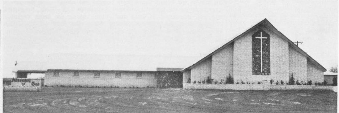
This beautiful new First Assembly in Yukon, Okla., which is constructed of white brick, has a sanctuary which seats 400.
