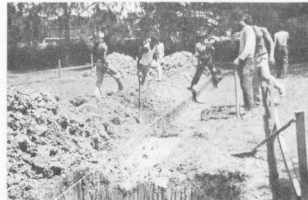
Foundation is laid.
