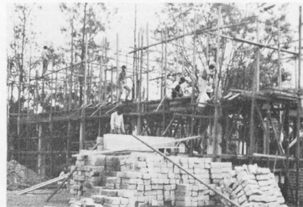
Administration building rises.
