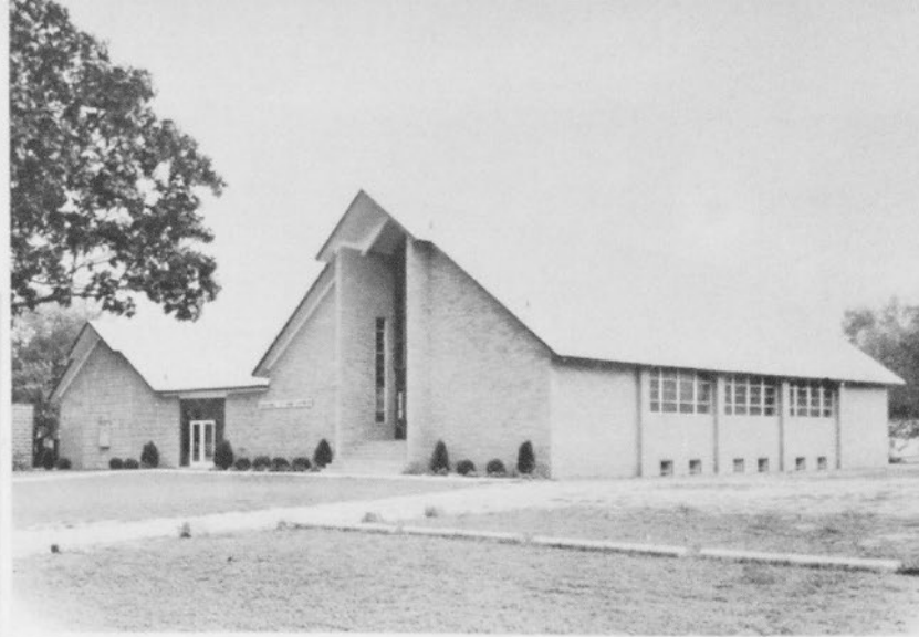
▲ PLYMOUTH, MICH.—Pastor John Walaskay and congregation dedicated a new sanctuary seating over 300 at the Assembly of God on September 27, 1964. An additional 75 can be seated in the balcony and another 30 in the choir area. The 50-by-80-foot addition with full basement is joined to the original church by a breezeway. The building is of laminated arch construction with buff brick veneer over cement block.
