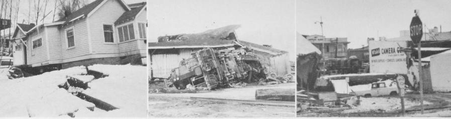
LEFT: Many homes in Alaska were ruined by the gigantic upheaval of the Good Friday earthquake. CENTER: This 79-ton Diesel engine at Seward, Alaska, was thrown 125 feet from the tracks and destroyed. RIGHT: On Fourth Avenue, Anchorage, the pavement suddenly dropped as much as 20 feet, breaking buildings in two.
