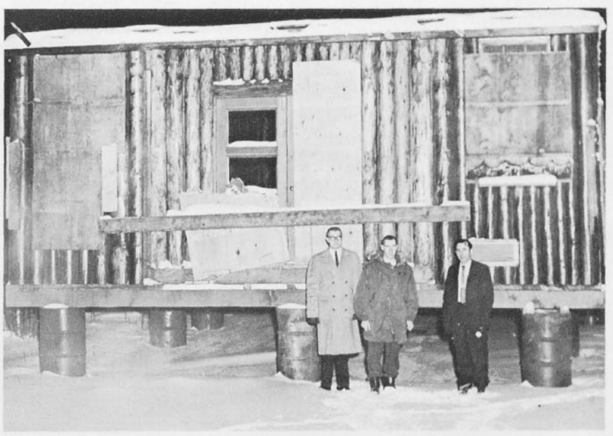
This building, formerly the church at Fairbanks, will be moved and set up at Nenana. The Fairbanks Assembly is building a new church.
