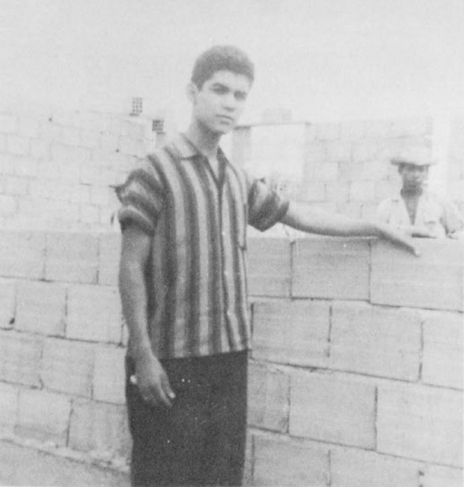
Venezuelan Bible school student Ramon Bejarano is thrilled to see the new building going up.
