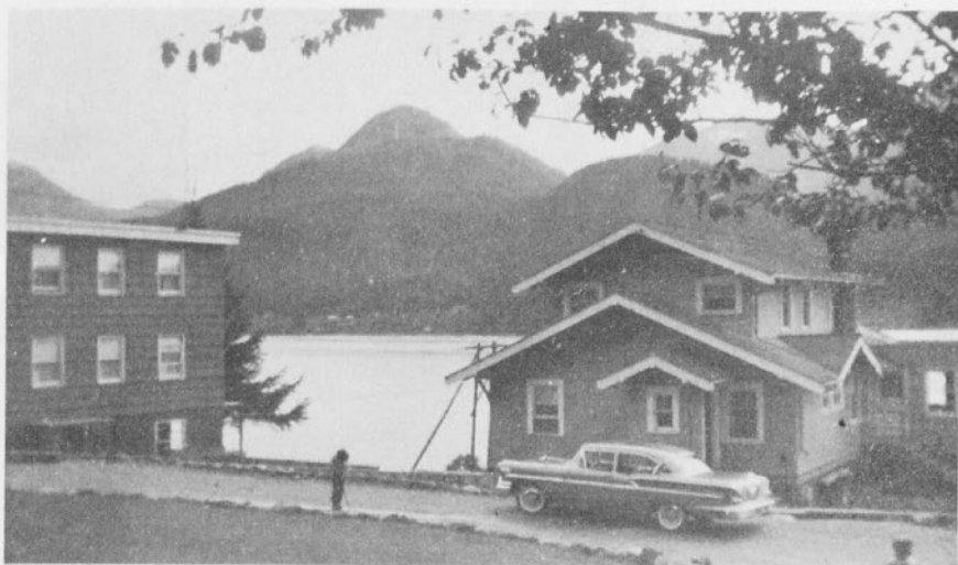
This summer scene shows the administration building of the Juneau Children's Home at the right; the dormitory appears at the left.
