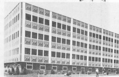
A 654-seat radio broadcast auditorium is located at the Pentecostal Assemblies of God headquarters building in Chicago.
