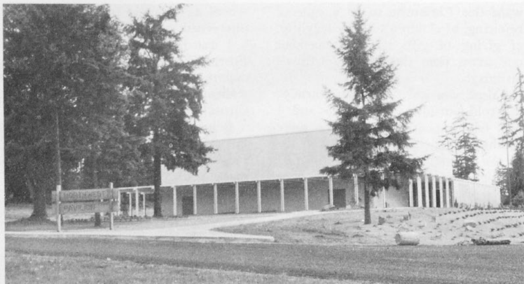
New Northwest Pavilion on the campus of Northwest College, Kirkland, Wash.
