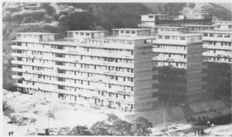
Seven-story government tenements like these house about 3,000 people per block in Hong Kong.
