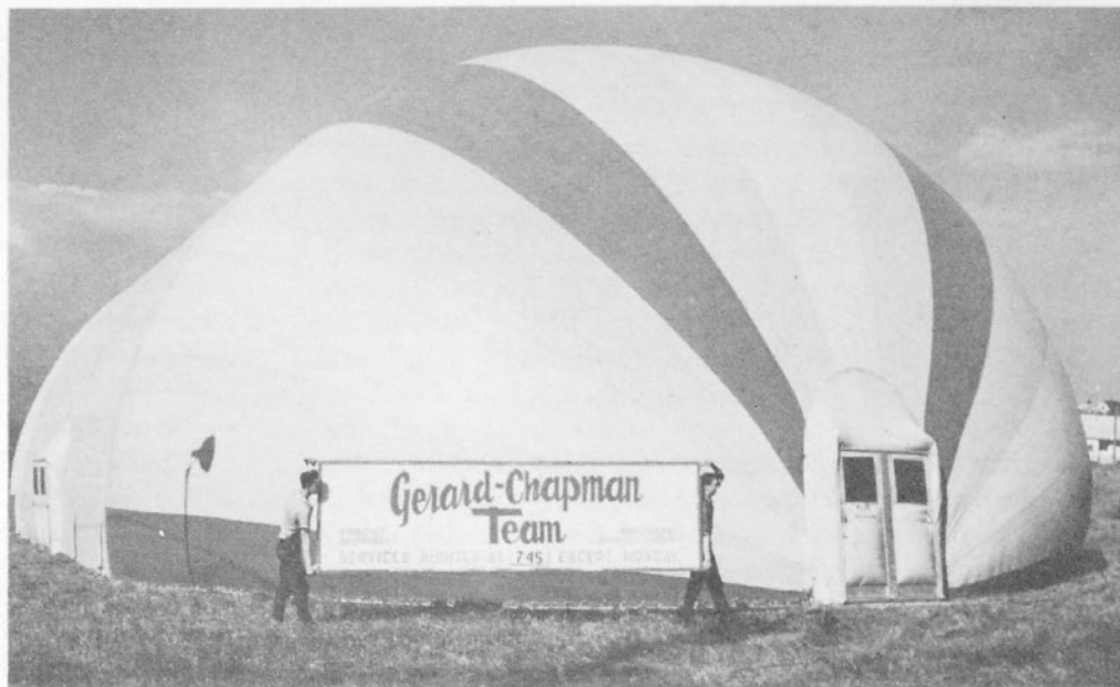
This "airatorium," which replaces the old-fashioned canvas tent, is maintained by air pressure.
