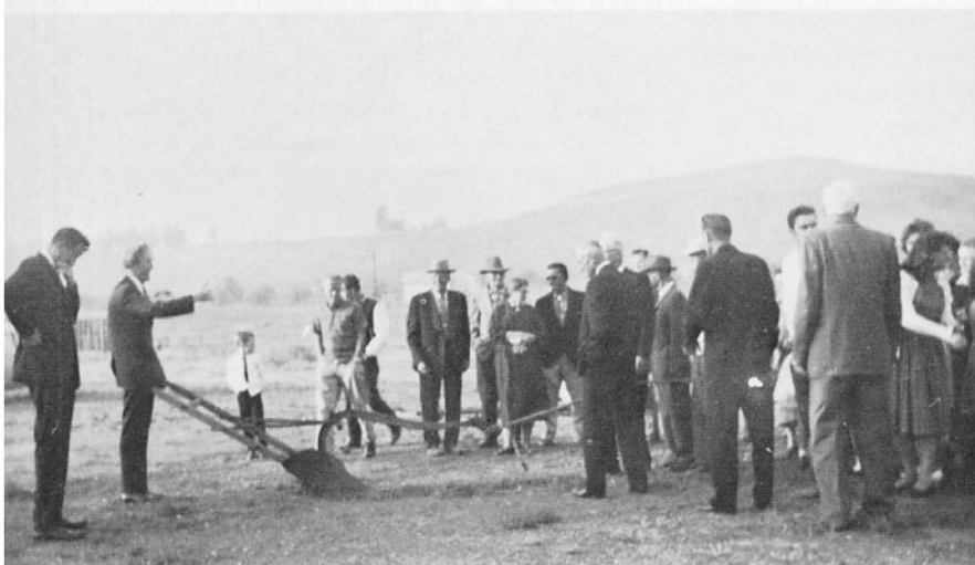
ELSINORE, CALIFORNIA—A man-powered plow was used at the ground-breaking of the new Elsinore Assembly of God on November 4, 1962. While the pastor guided the plow, the board and church members all pulled on a long rope to make the ceremony very impressive and meaningful. D. F. Ferguson, sectional presbyter, stands at the left while Pastor L. L. Ammons exhorts the congregation to "keep pulling together."
