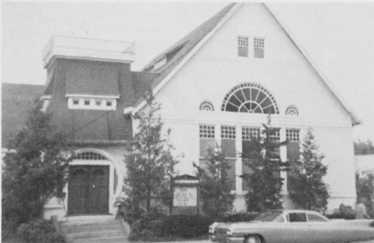
GREENFIELD, INDIANA —This new home of the Assembly of God in Greenfield, purchased last September, will seat 175 and it has an overflow annex. The Sunday school has increased since moving to the new location. The church was begun in 1954 by C. W. Syler. James F. Flower has been pastor since 1956.
