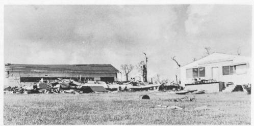
The church was moved 30 feet from its foundation and the house was badly damaged.
