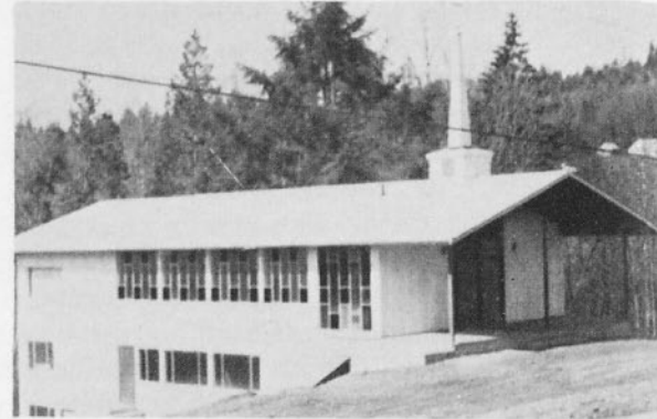
LONGVIEW, WASHINGTON—Pastor R. J. Mitchell and congregation of Columbia Heights Assembly recently completed this building. The church is five years old.
