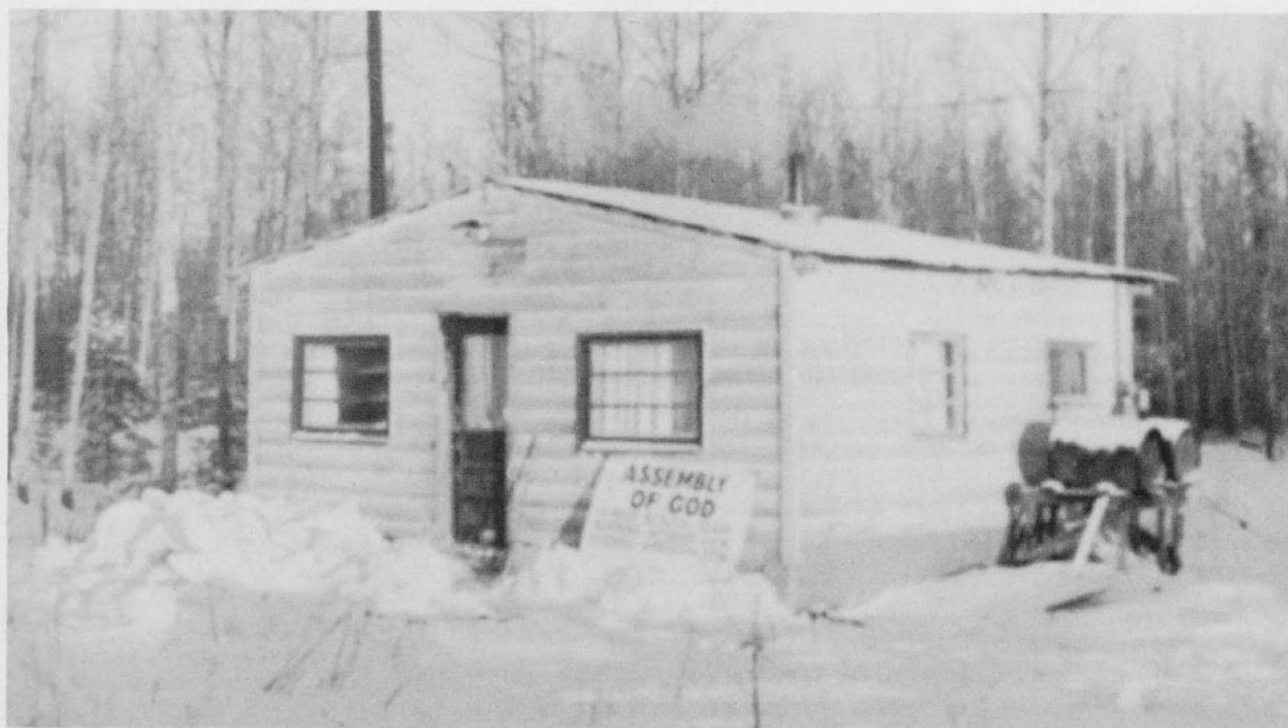
Parsonage at Delta Junction, Alaska, which serves as the church building until the small congregation can build a church on this property.
