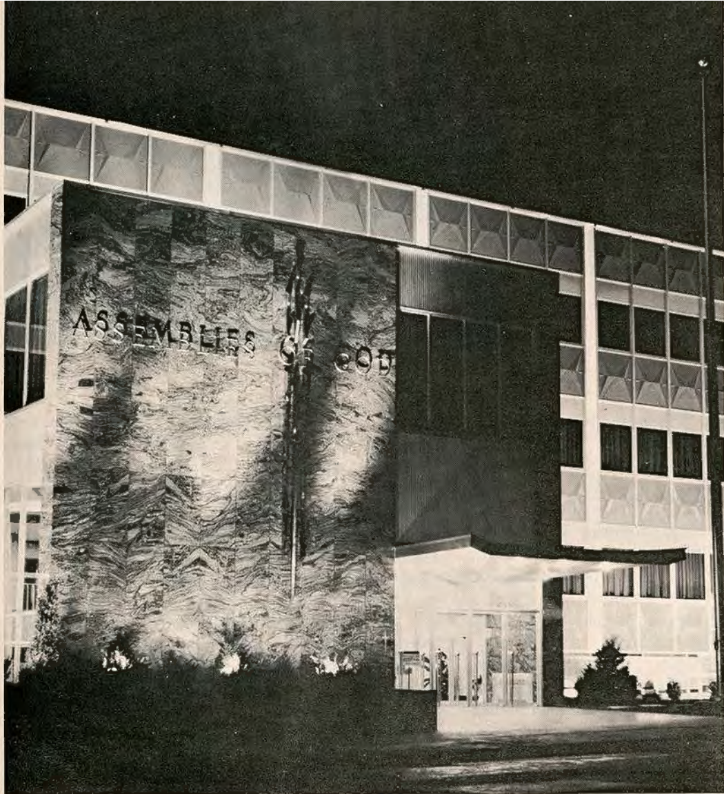
The long expanse of the new international headquarters building is broken by this handsome foyer which is encased in rainbow granite.
