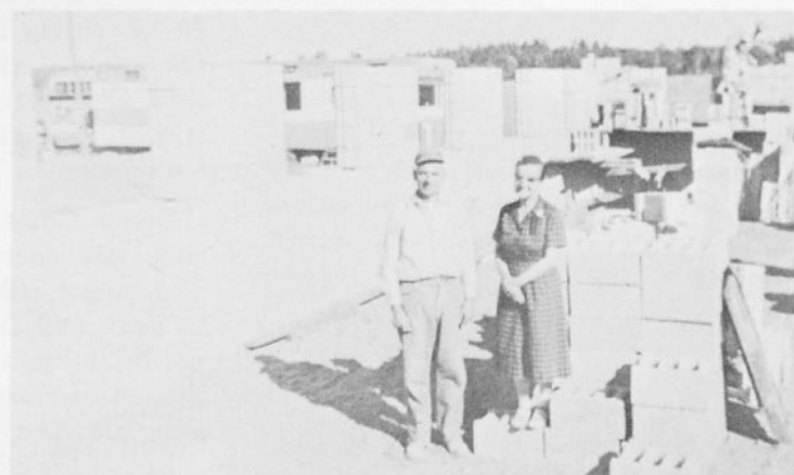
Mr. and Mrs. Norman Rehwinkel, missionaries at Keshena, Wis. stand beside the new church building being erected.
