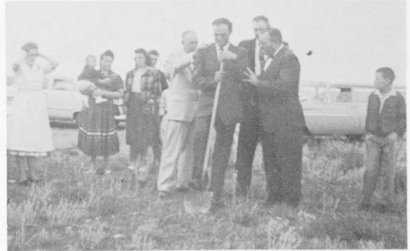
J. E. Gerrard holds the shovel for the ground-breaking service while Brothers Beard, Ventling, and Little pray with him.
