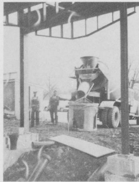
Mixing trucks emptied the concrete into a huge iron bucket.
