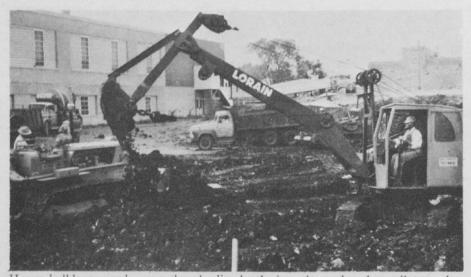
Heavy bulldozers and scoop shovels dig deeply into the rocky clay soil to make room for footings and basement.
