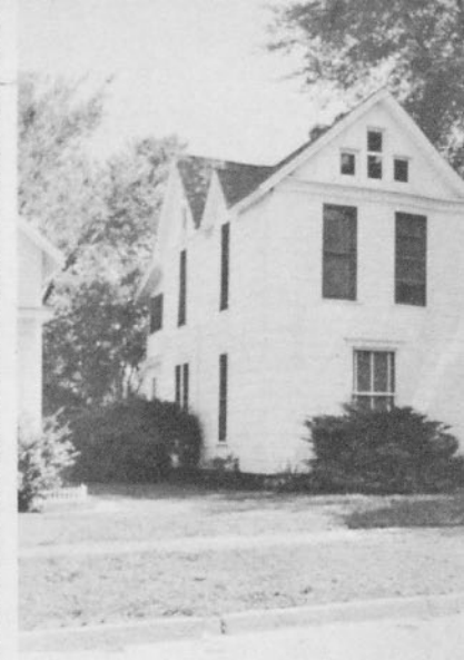
One of houses to be razed.
