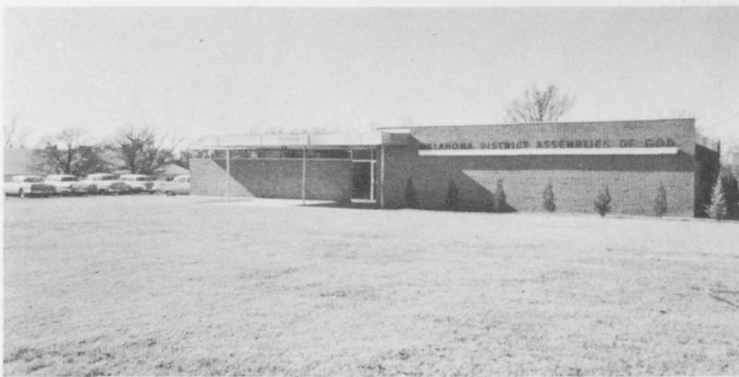
Pictured above is the beautiful new district office building for Oklahoma. Located on ten acres in Oklahoma City, it is 52' x 80' and contains 4,000 square feet. There are offices for six district officials and their secretaries, a reception room, conference room, and two general work rooms. The building is air conditioned throughout and is of modern design with masonry of pink Roman brick. The total cost was $61,000 and the building is debt free.
