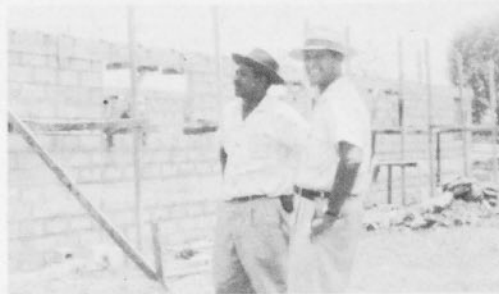
Enrique Suarez, district superintendent, and contractor survey the unfinished building at the Dominican Republic Bible School
