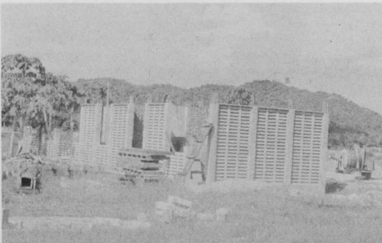
Louvered block walls of the new church for the Orphanage
